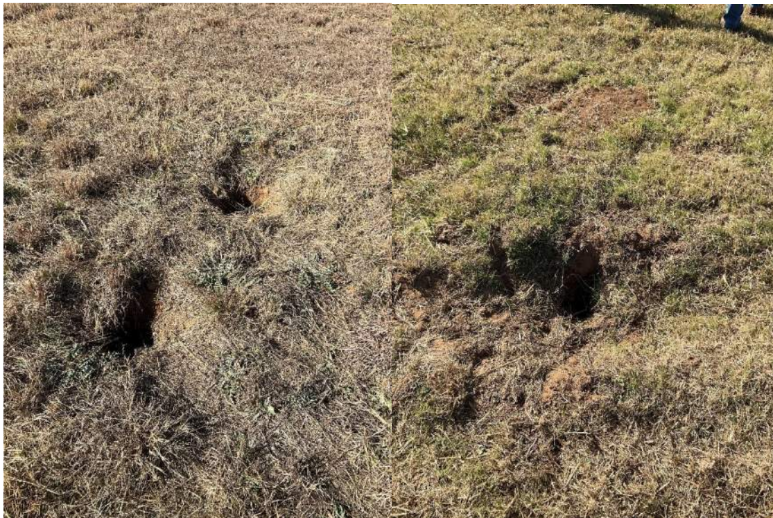
Figure 2: Sink holes over drainage pipes
