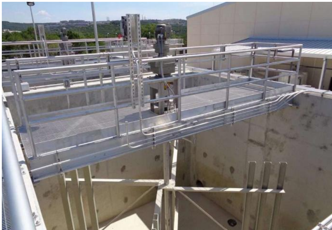
Figure 2-4. Typical Vertical Paddle Wheel Flocculator
