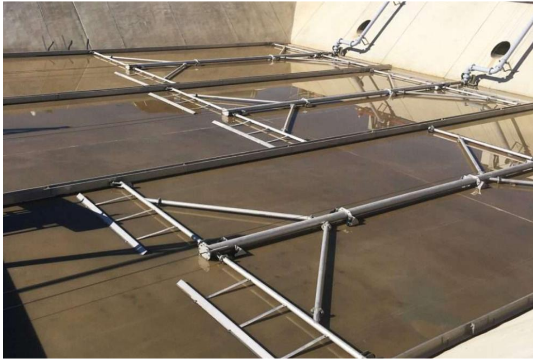
Figure 2-6. Typical Hose-less Sludge Removal System
