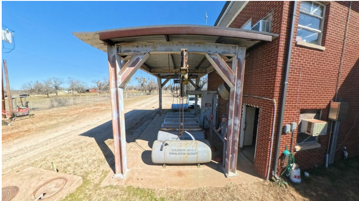
Figure 3-5. Chlorine Tanks
