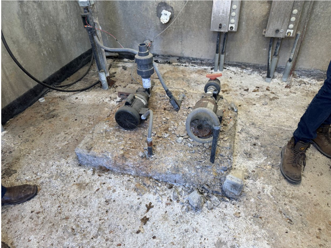
Figure 3-4. Chemical Storage Building Floor
