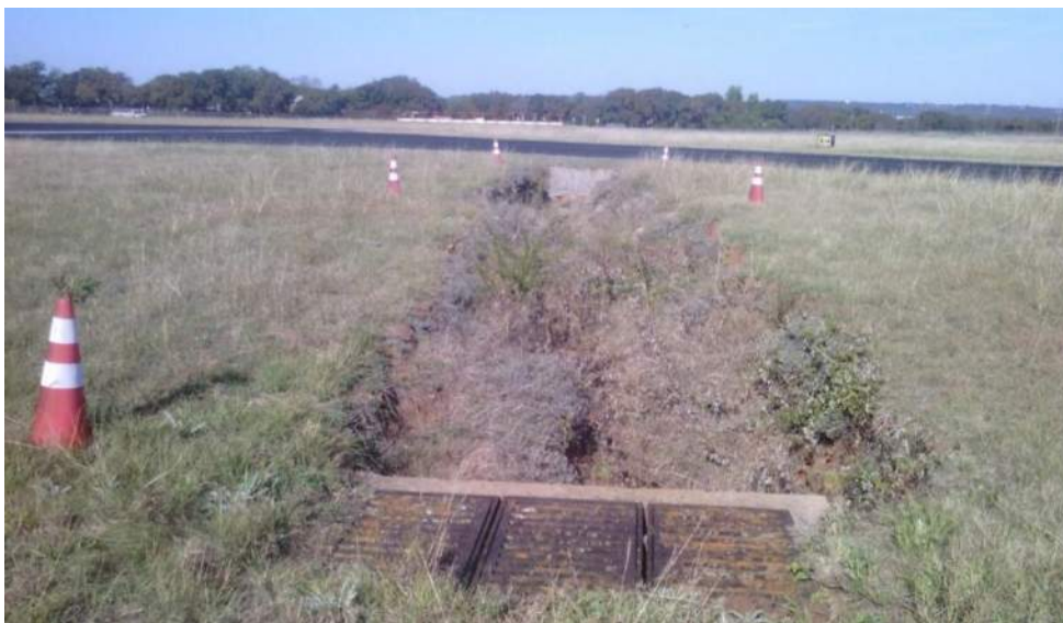
Figure 3-10. Collapsed Culvert
