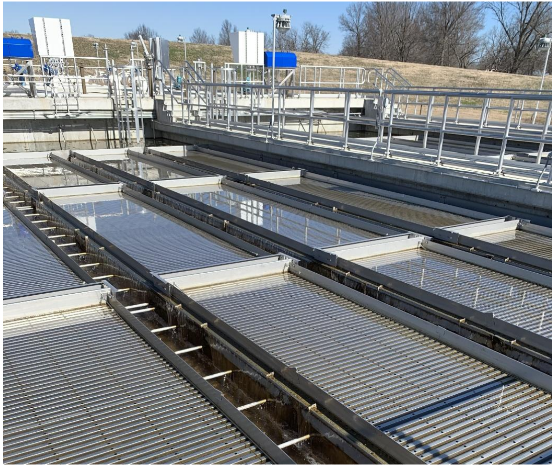
Figure 2-5. Typical Plate Settler System
